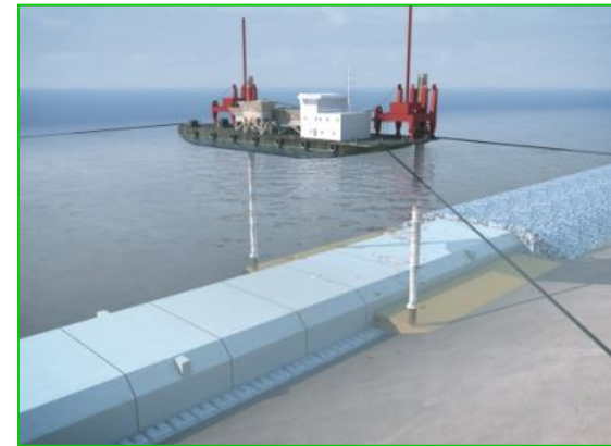
Lock backfilling
