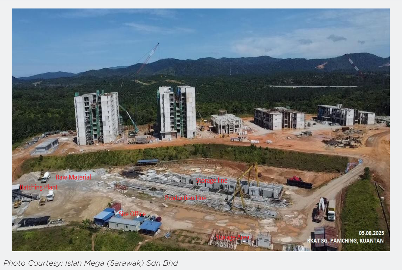
Temporary precast concrete casting yard layout:
